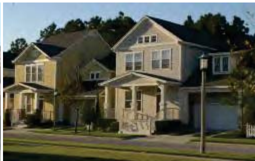
Figure 29 – Attached garages must be a natural extension of the design, massing and materials of the main dwelling
