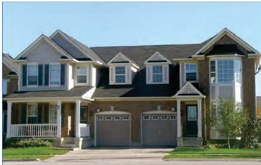
Figure 9: Semi-detached dwellings with attached garage that appear recessed through use of a projecting porch
