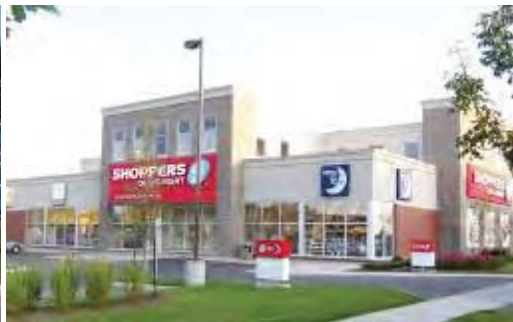
Figure 25: Non-street facing buildings can provide visual interest through architectural detailing like the main façade
