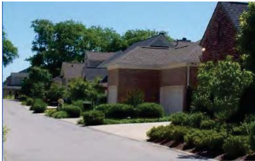
Figure 26: Lane-based garages should be designed to provide an attractive visual environment
