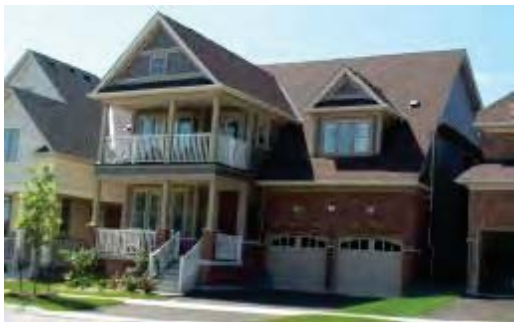
Figure 28: Garage are setback behind the mail wall face or the front porch
