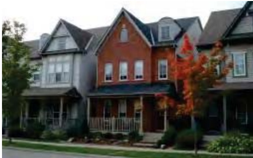
Figure 7: Entrance features may encroach into required set-backs
