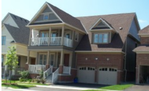
Figure 28: Garage are setback behind the main wall face or the front porch
