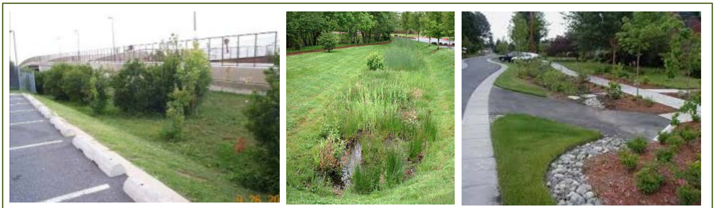
Figure 4-4: Filter Strips for Pre-Treatment for Parking Lot Runoff (Left, Source: CWP) or Prior to Entering Another Stormwater Management Facility (Middle, Source: Minnesota Stormwater Manual. Right, Source: Seattle Public Utilities).
