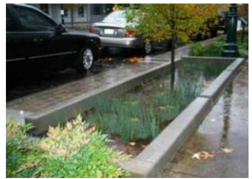
Extended tree pits (Source: TRCA) in Portland, Oregon.
