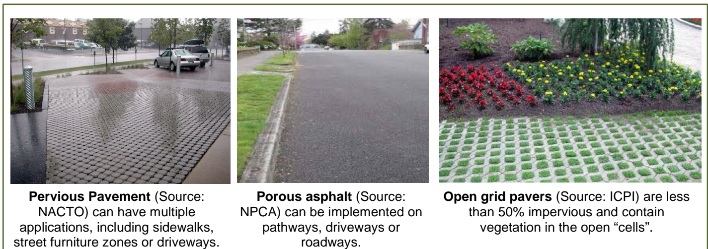
Figure 4-8: Permeable Pavement Options
