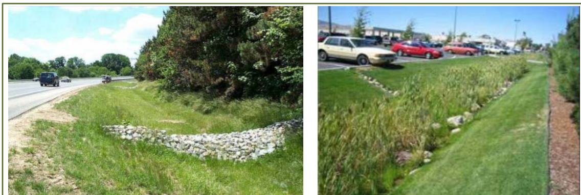
Figure 4-6: Enhanced Grass Swales Adjacent to Major Roads or Parking Lots to Increase Pollutant Retention and Decrease Flow Velocity (Left, Source: Delaware Department of Transportation, Right, Source: CVC).
